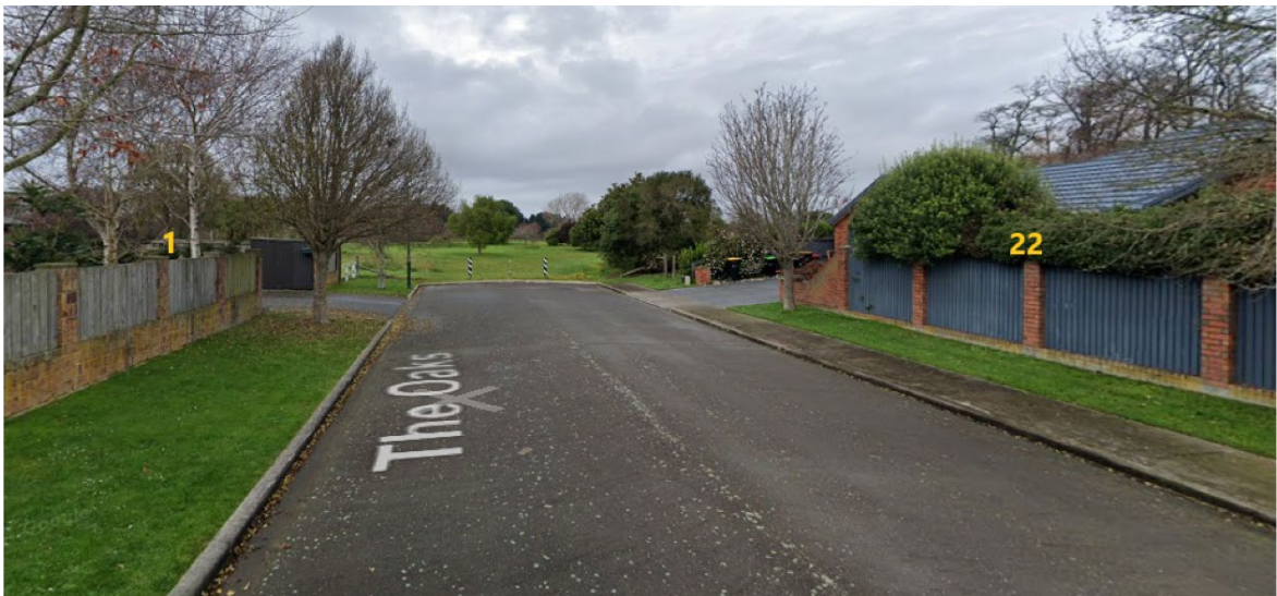
Figure 2. Decommissioning of The Oaks
