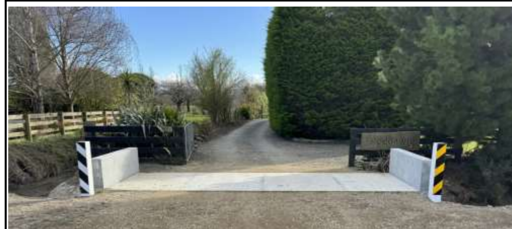
Woodfields Road Drainage Improvements Culvert Upgrade
