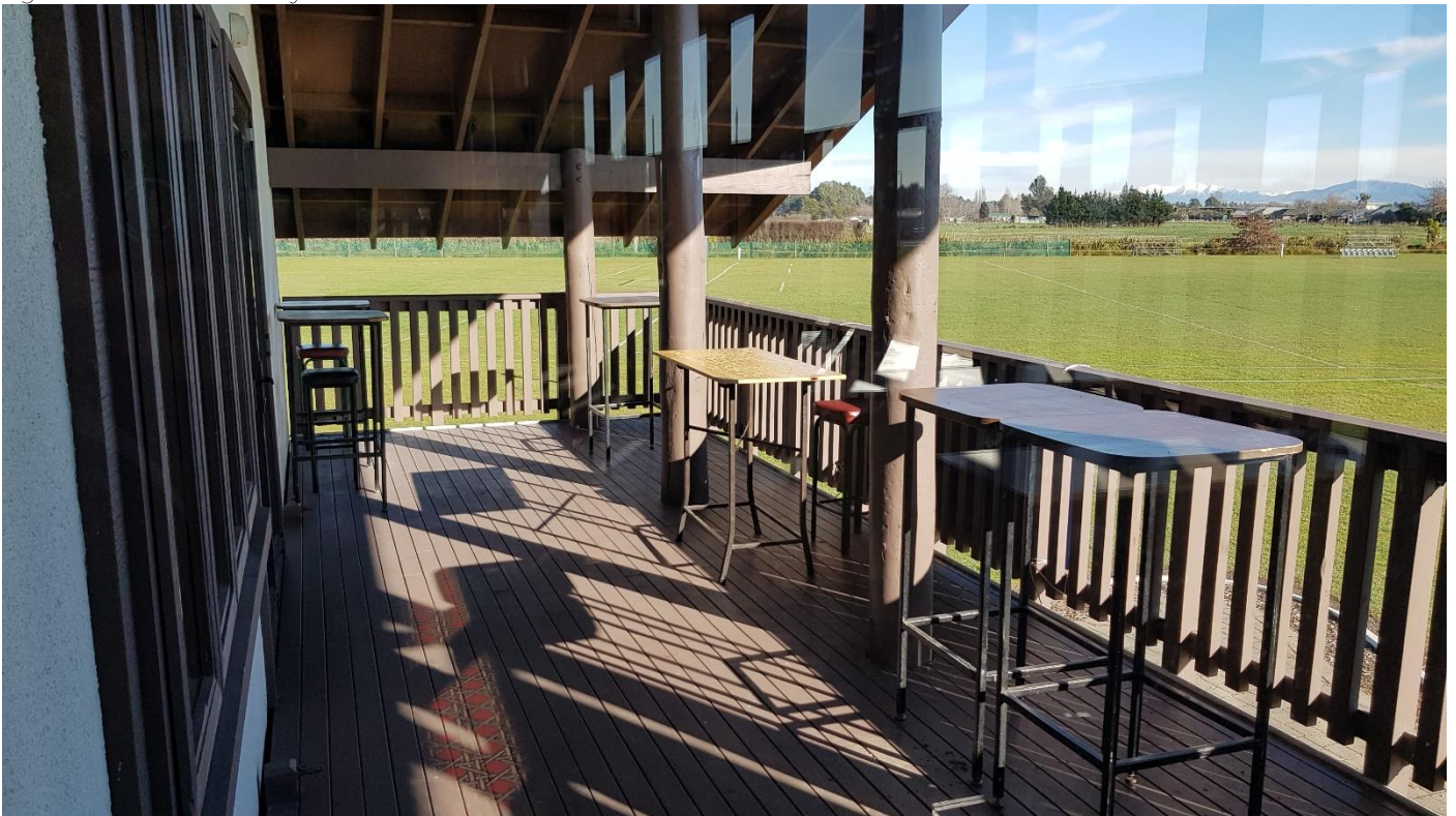
Figure 7. First Floor Balcony
