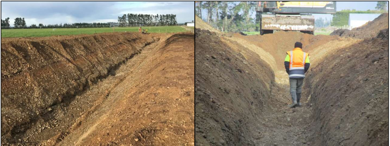
Figure 2 Overview of the empty trench
