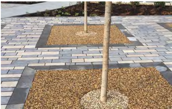
Figure 3. Tree pit, surrounded by pavers (Source: https://www.geveko-markings.com/cases/stunning-tree-pits-with-geopavex/ )
