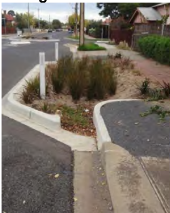
Figure 1. Roadside Rain Garden (Source: https://www.watersensitivesa.com/wp-content/uploads/Plant-Species-Selection-in-Stormwater-Biofilters-Wetlands_S-Kennedy_Handouts.pdf )
