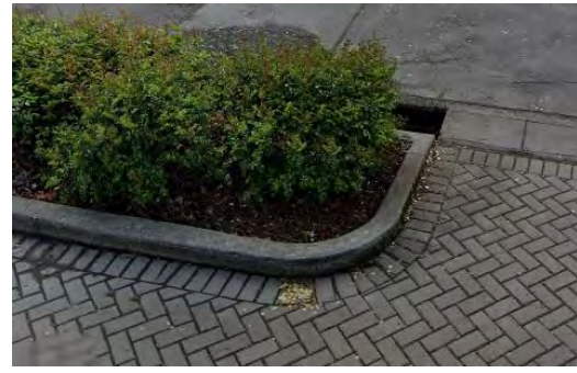
Good kerb &amp; channel
