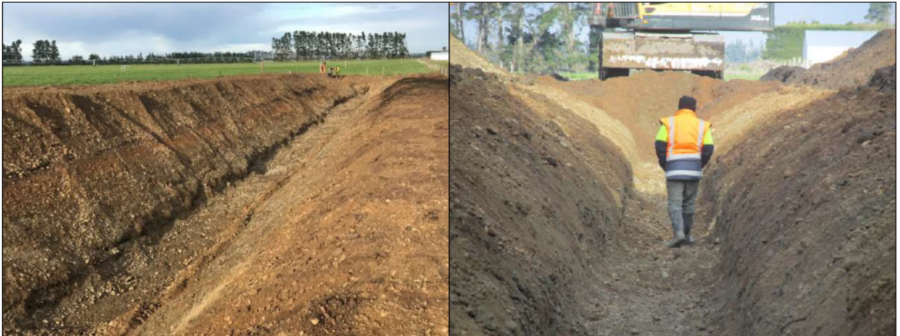
Figure 2 Overview of the empty trench
