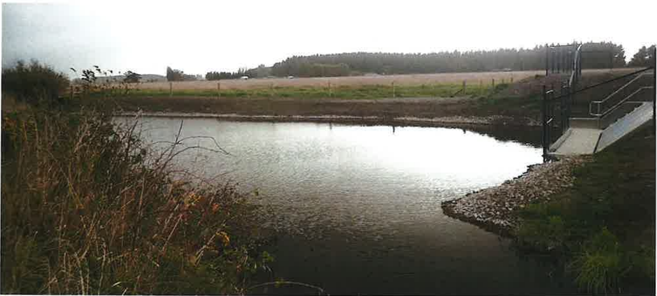
Figure xiv. Looking at the true left (east) bank of McIntosh Drain, upstream of the tide gates. The graded bank around the pumphouse will provide inanga spawning habitat when planted.
