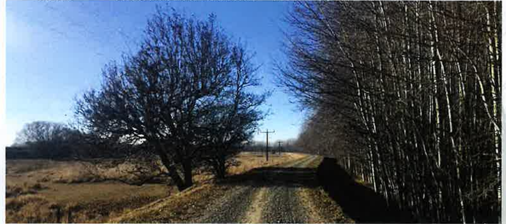
BELOW: Stopbanks are a vital piece of flood protection infrastructure used along the Rangiora Reach.
