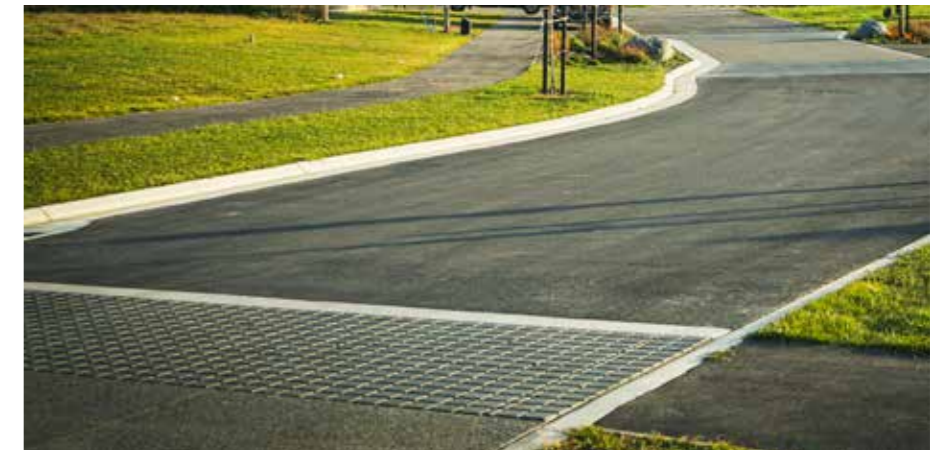
PROVISION OF CROSSING FACILITIES AND MATERIAL CHANGES AS TRAFFIC CALMING MEASURES
