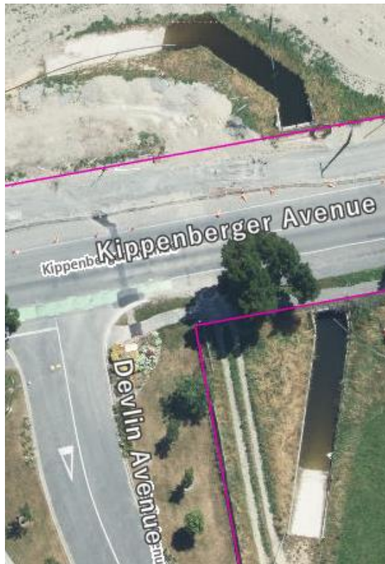
Figure 2: Aerial image showing natural groundwater level with pump off.
