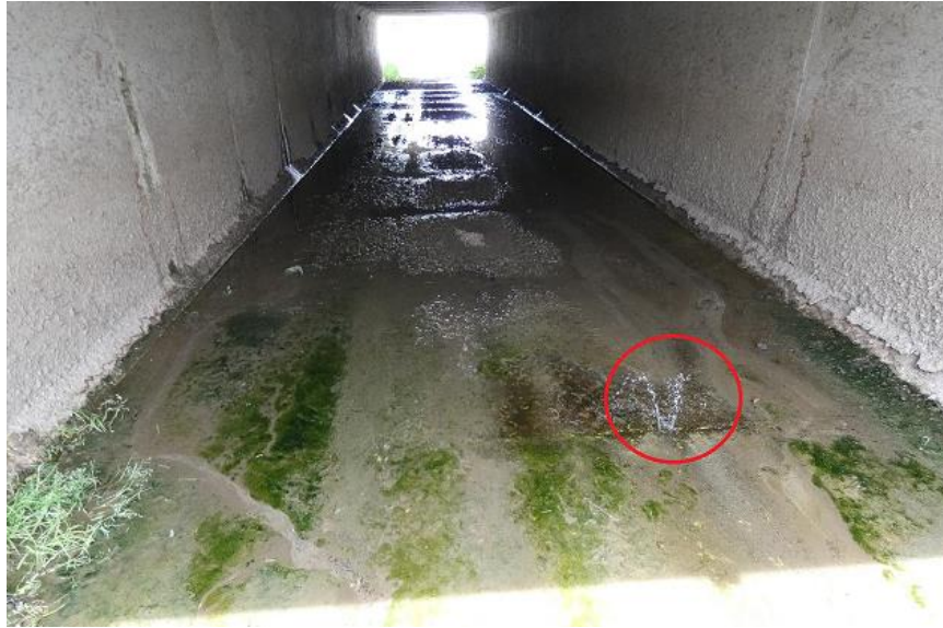
Figure 3: Water spouting through floor join (red circle) and algae growth, November 2021
