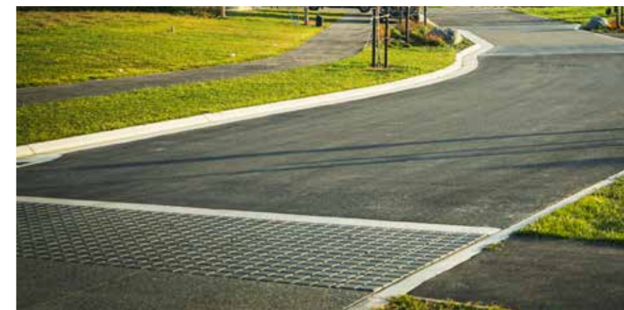
PROVISION OF CROSSING FACILITIES AND MATERIAL CHANGES AS TRAFFIC CALMING MEASURES
