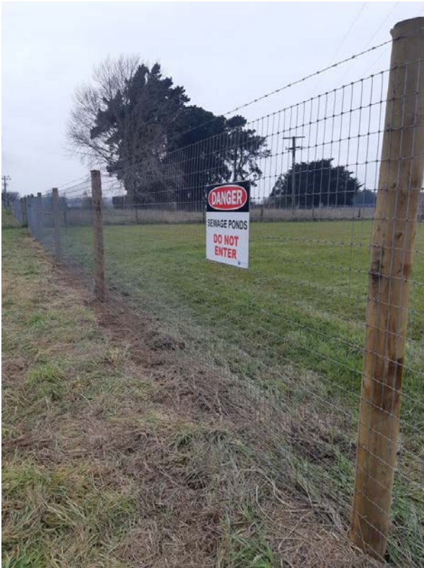
Figure 1: X-Fence, barbed wire and signage installed at the Rangiora WWTP site
