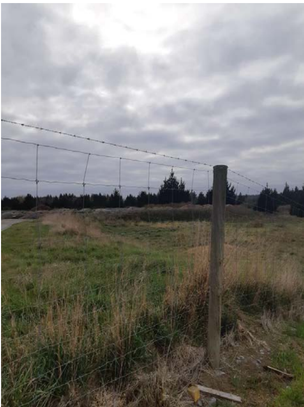
Figure 2: Barbed Wire installed at the Kaiapoi WWTP
