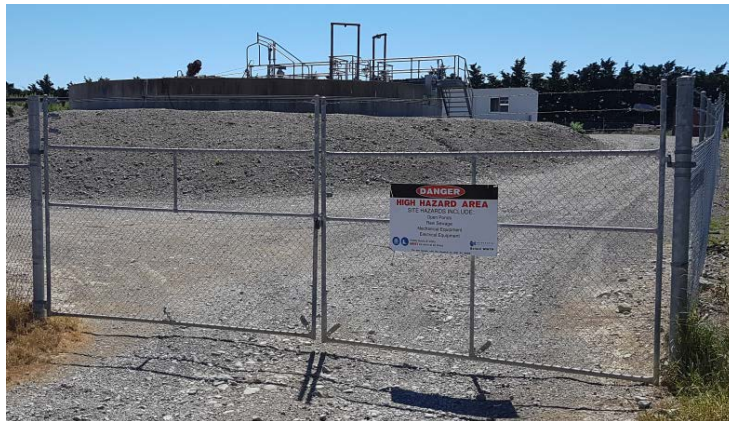
Figure 2.2: Security Fence (Oxford WWTP)
