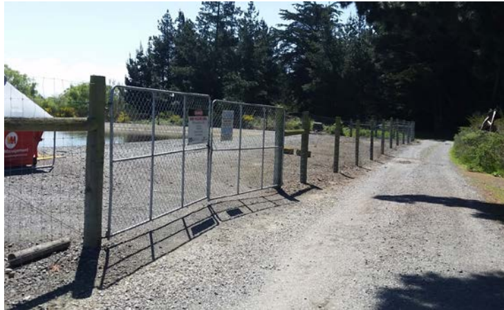
Figure 2.1: Deer Fence (Waikuku WWTP)
