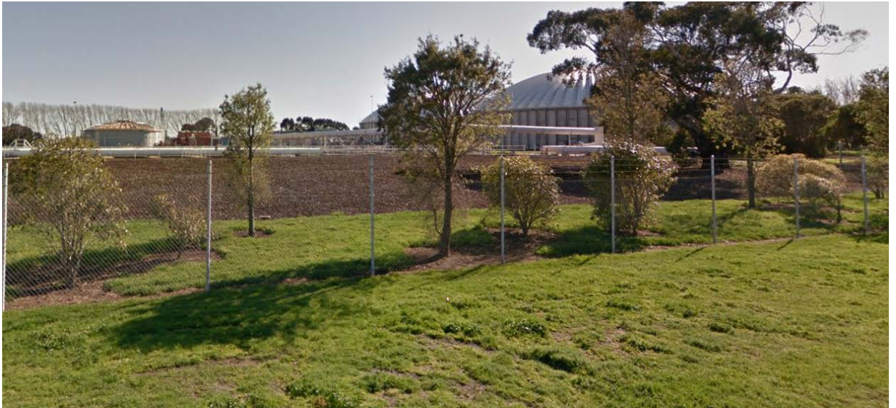
Figure 3.3: Bromley WWTP Christchurch – Security Fence
