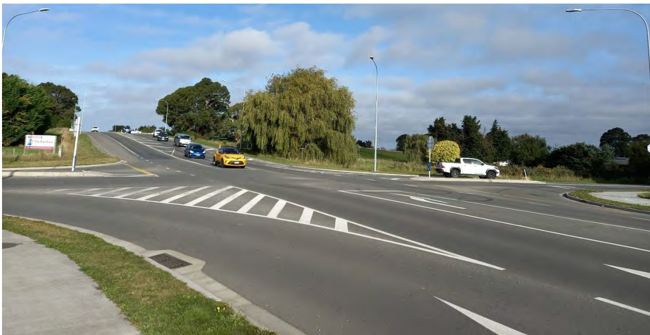
Figure 4 Current Ohoka Road/Island Road intersection – view for the southwest corner
