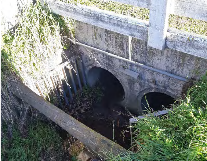
Figure 3: Ashley Street Culvert Outlet
