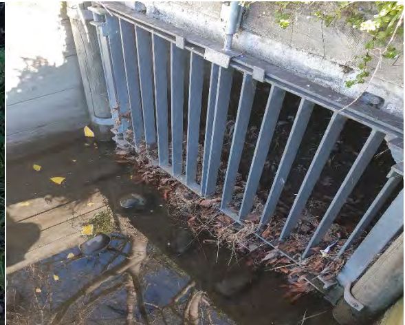
Figure 5: Edward Street Culvert Outlet
