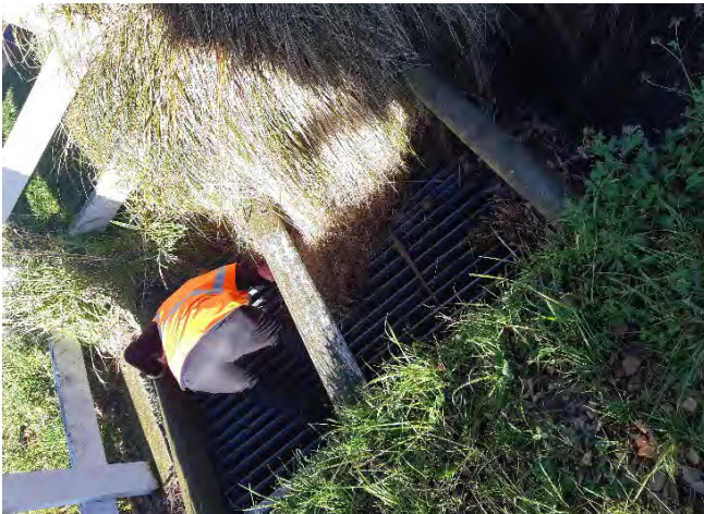
Figure 4: Edward Street Culvert Inlet
