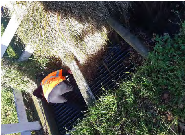
Figure 4: Edward Street Culvert Inlet
