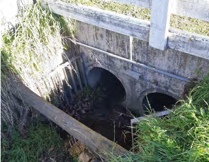
Figure 3: Ashley Street Culvert Outlet
