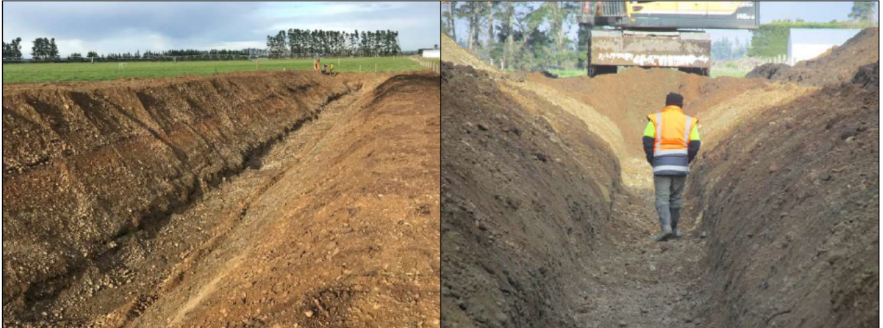
Figure 2 Overview of the empty trench
