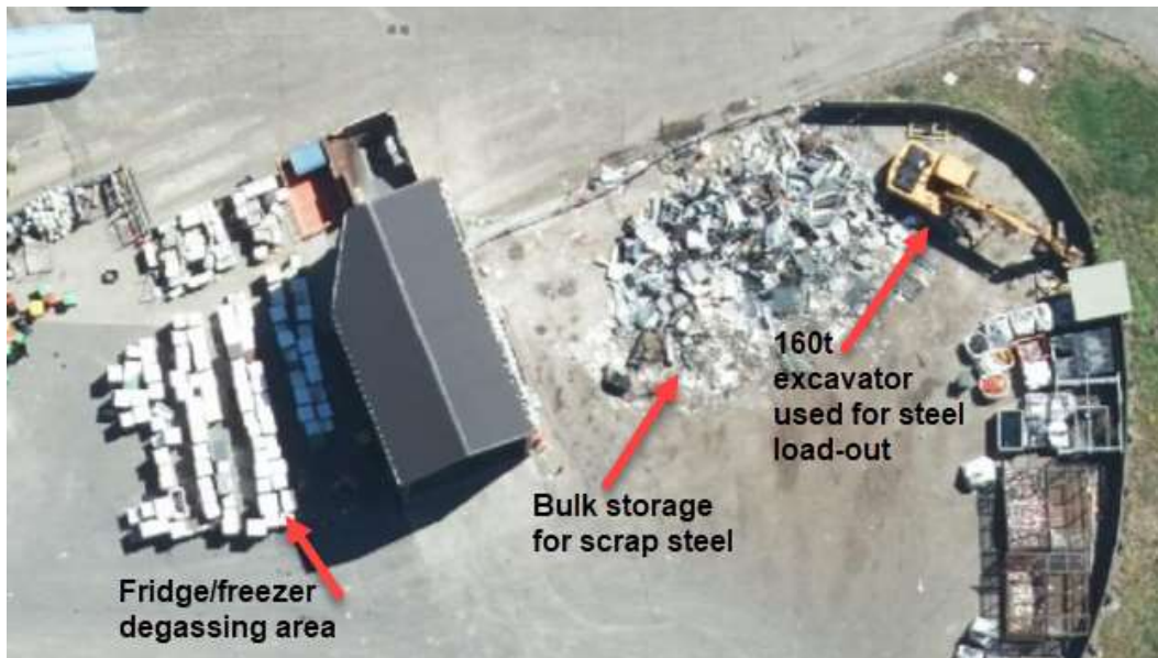
Figure 3.2: Scrap Steel and Fridge/Freezer storage area beside shed
