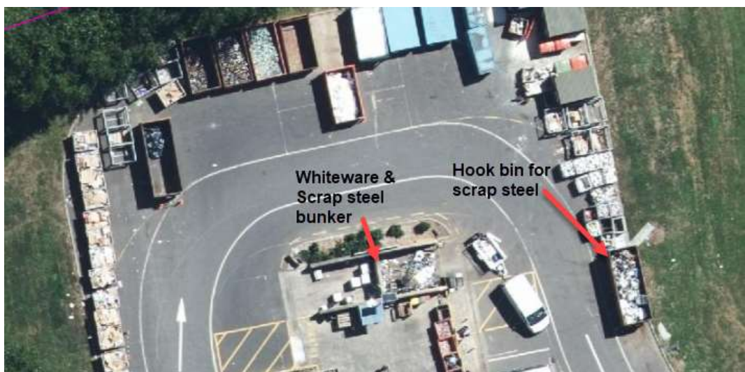
Figure 3.3 Scrap Steel bunker and hook-bin
