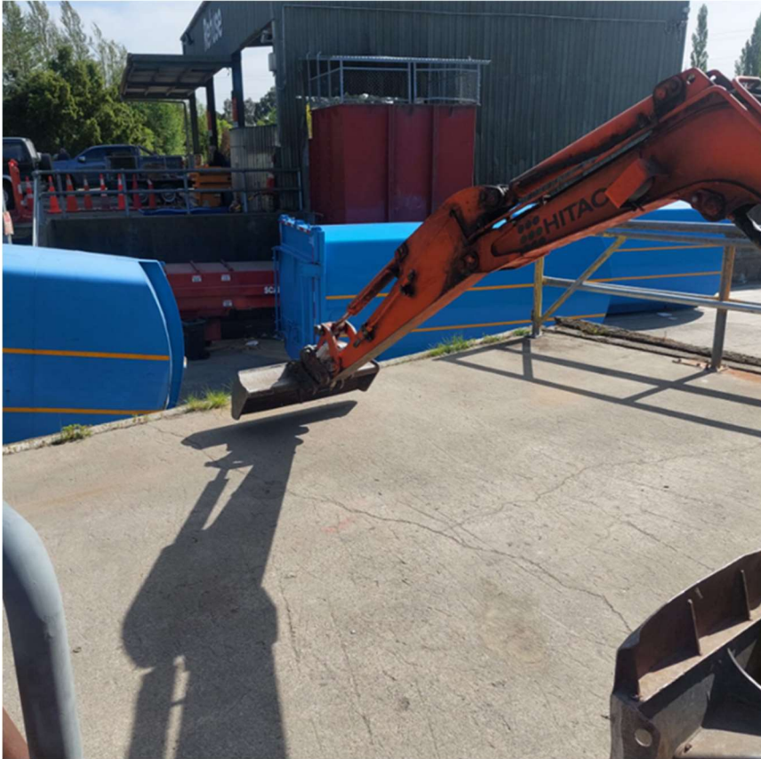
Figure 4.3: Use of Excavator to push steel over edge into container-trailer below.
