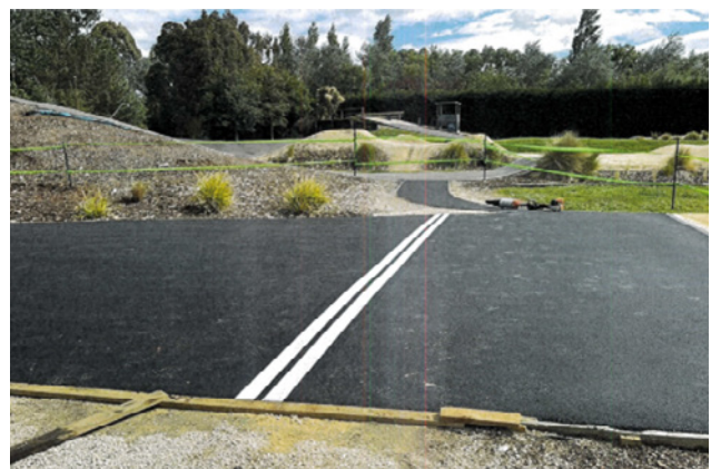
Asphalting at the Rangiora BMX track
