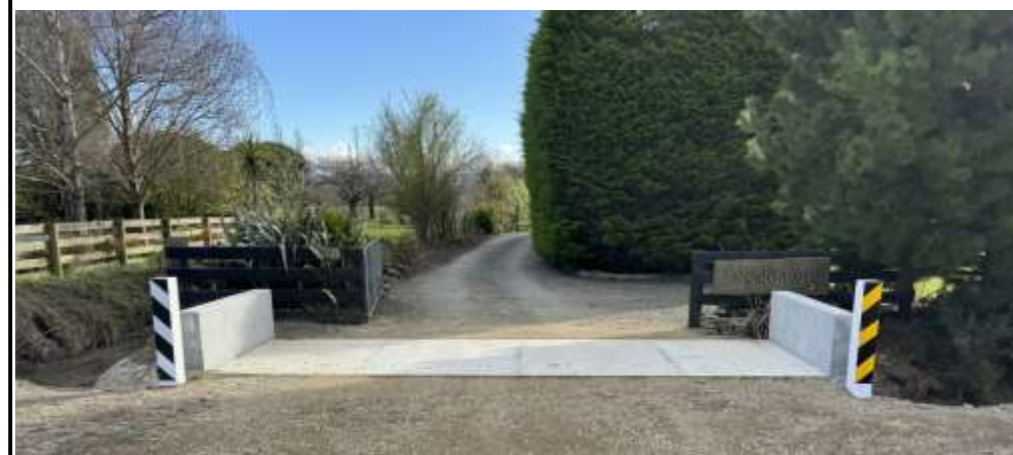
Woodfields Road Drainage Improvements box culvert install
