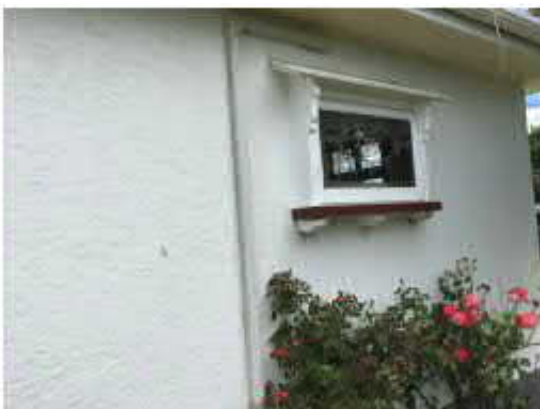
Figure 3: Plastered pre-1940s weather board dwelling.
