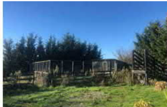
Photo 4. Cattle yards and garden shed
