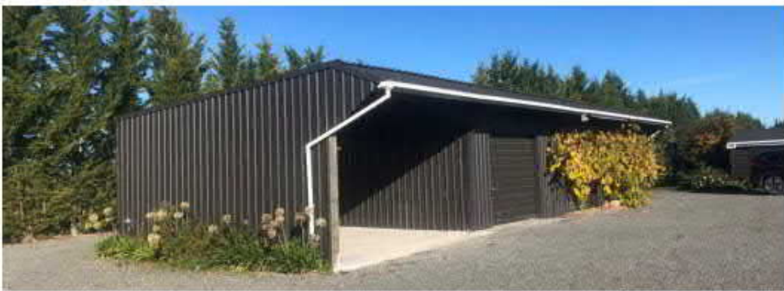
Photo 2. View of the garage and shed located to the southeast of the residential dwelling
