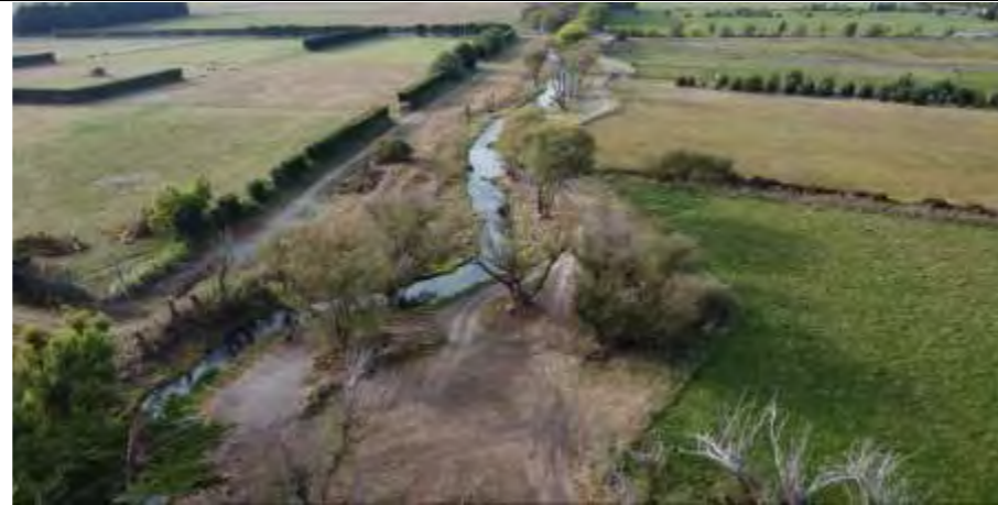
Cam River Maintenance Works
