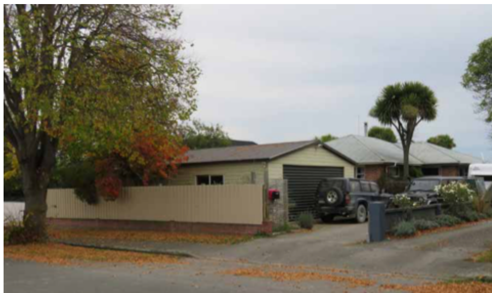
Photo 1: Garage in front garden restricting views between the street and the house, Rangiora
