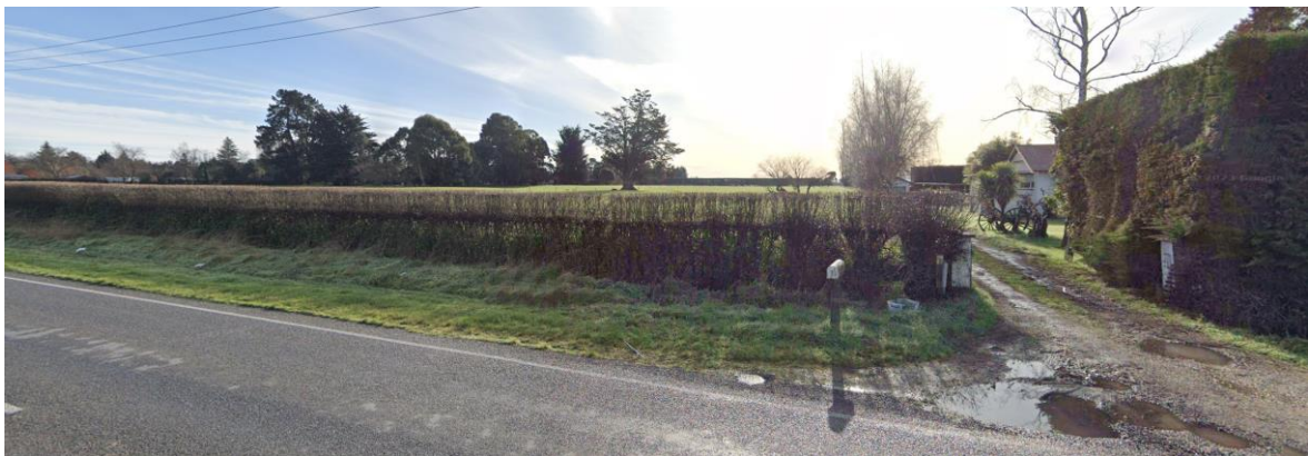
Figure 25. View from outside the south-eastern corner of the site from Rangiora Woodend Road, opposite the old weatherboard farmhouse at 494 Rangiora Woodend Road, as well as the mature trees (exotic) surrounding the existing dwelling at 518 Rangiora Woodend Road (the Site's) curtilage (Google, 2023b)
