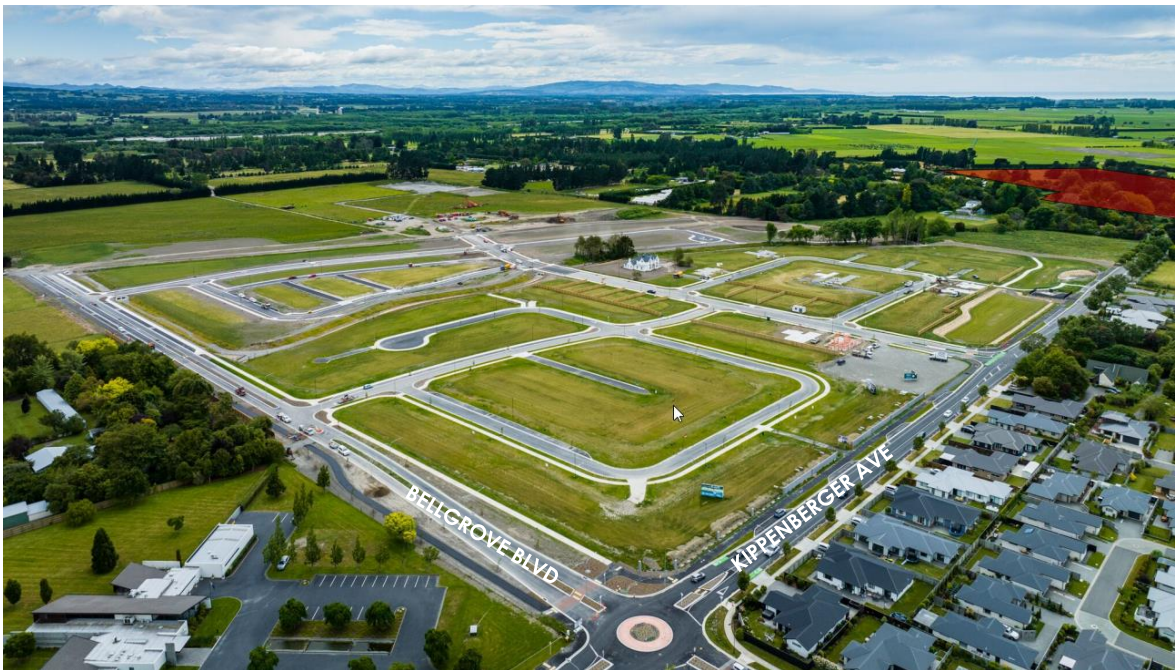
Figure 7. Aerial view of Bellgrove Stage 1A (image: https://www.facebook.com/BellgroveRangiora/ ) with the Site overlaid (indicative only)
