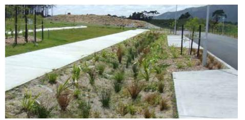
INCLUSION OF BIORETENTION SWALE TO CAPTURE AND TREAT STORMWATER RUNOFF
