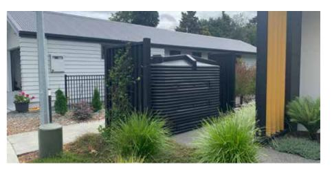
INTEGRATION OF RAINWATER TANKS TO REDUCE RUNOFF PEAKS AS WELL AS REDUCE MAINS WATER USAGE
