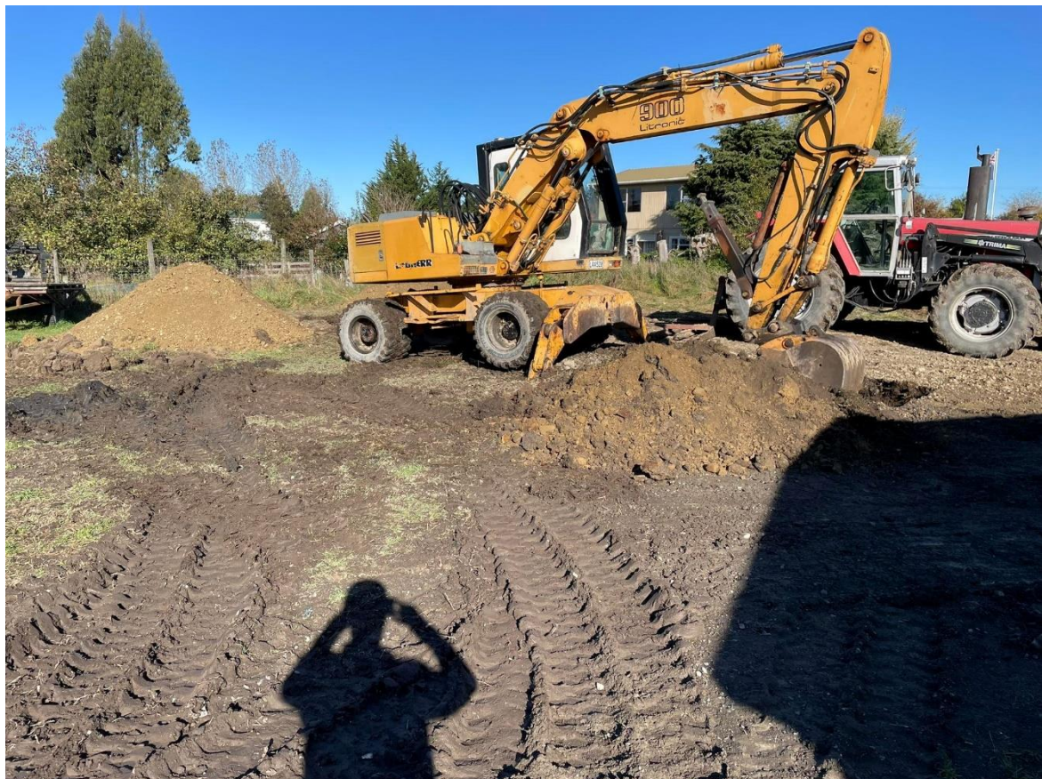
Figure 6: View of the digger used for test pits and the soil conditions (Looking Southwest)
