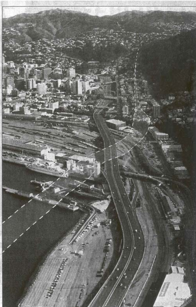
Figure 2 Newspaper article showing the line of the newly mapped Wellington Fault (looking south). The photo does not show the Fault Rupture Hazard Zone with the buffer. The article reflects effective communication between the WCC and the Dominion Post which has reported positively and discussed key issues such as building restrictions, valuations, public consultation and insurance. Source: Dominion Post, Wellington, 5 April 2003
