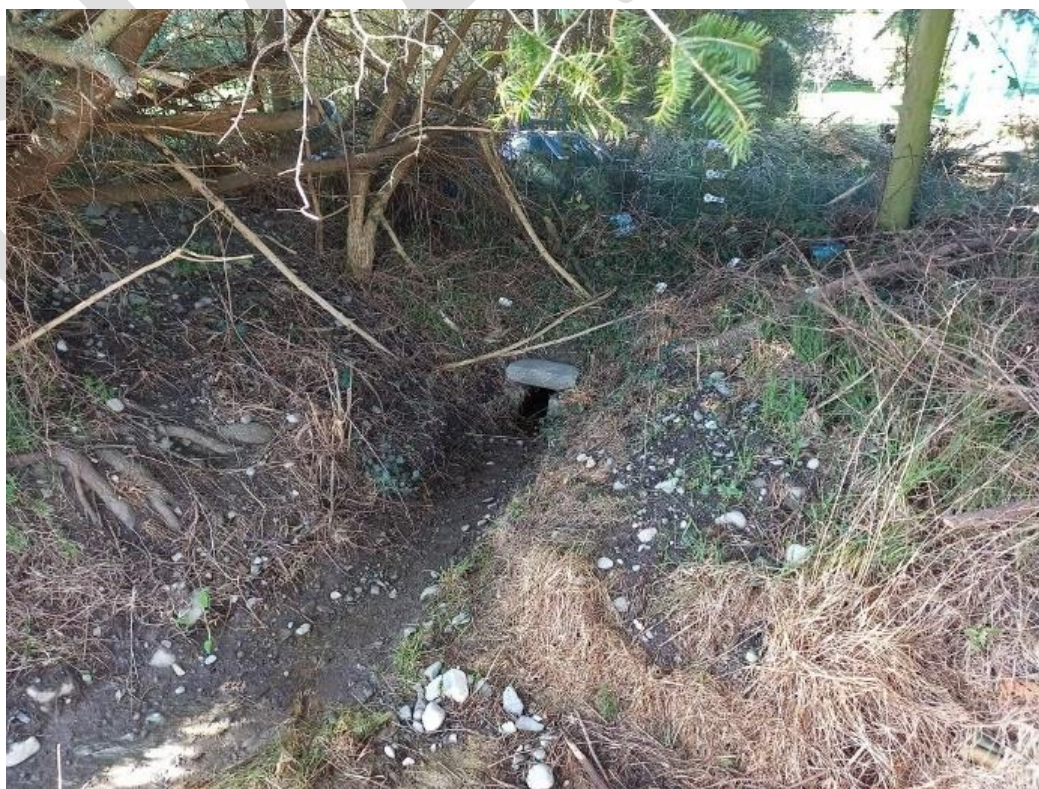
Figure 1: Swale Entrance into 55A Burnett Street
