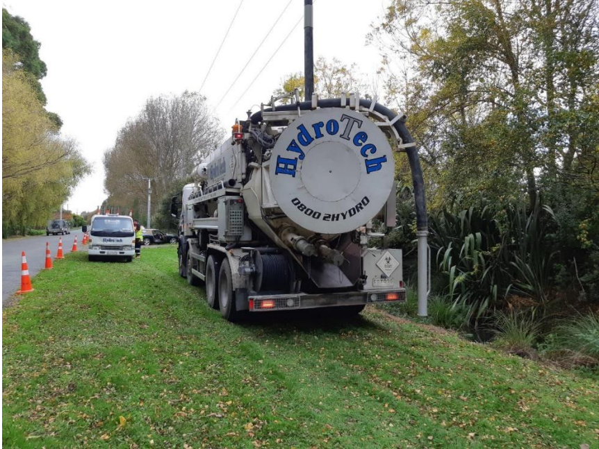
Figure 4 – The sucker truck that was used for the Greens Road sediment trap emptying trial
