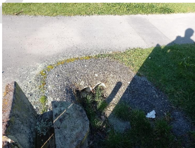
Figure 9: Piped Swale Outlet 53 Burnett Street
