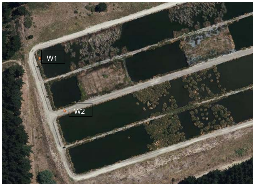
Figure 5: Midge emergence trap locations (red pins) of the two traps at Woodend Wastewater Treatment Plant during the summer and autumn of 2021-22.
