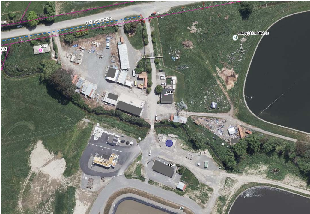
Figure 5: Recommended location of waste disposal bin location (purple dot) at Rangiora Wastewater Treatment Plant.
