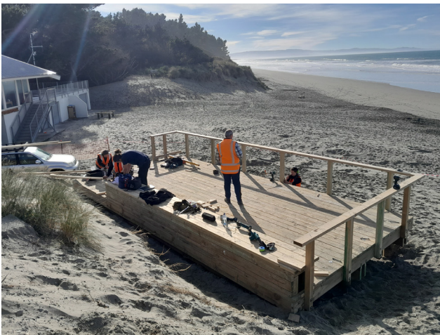
Progress on Waikuku Beach accessible platform
