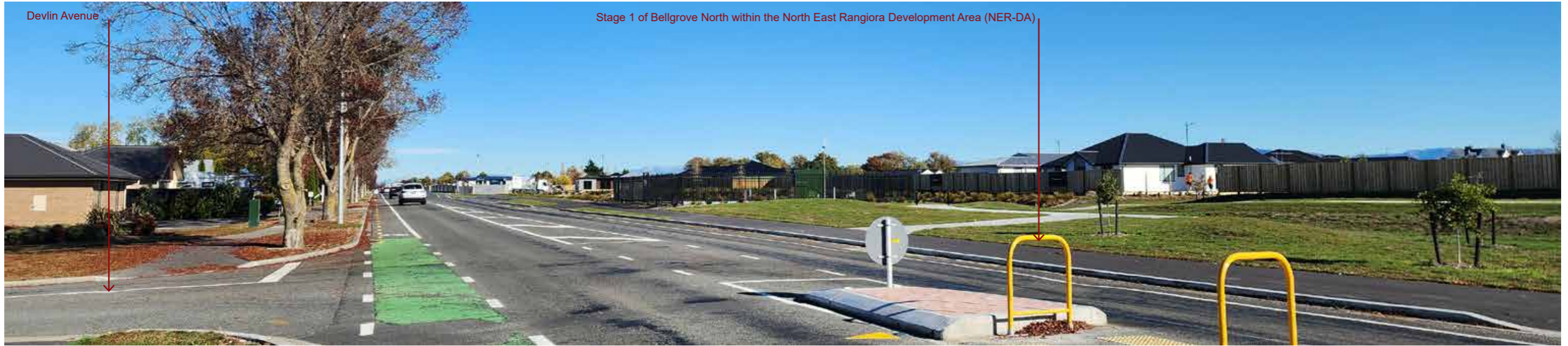
Site Photograph 5: Looking west along Kippenberger Avenue
