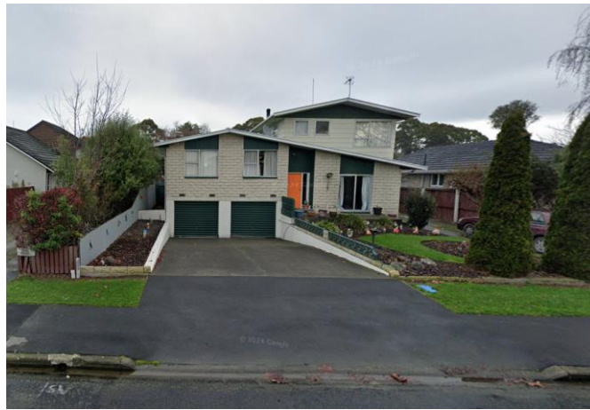
Figure 1 - 7 Aldersgate Street in Kaiapoi
