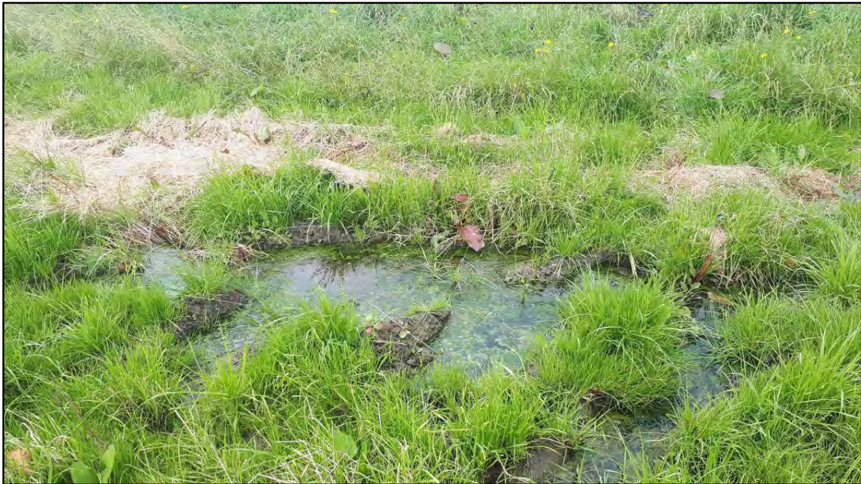
Figure 7. Surface ponding observed on 9 March 2022 by Environment Canterbury
