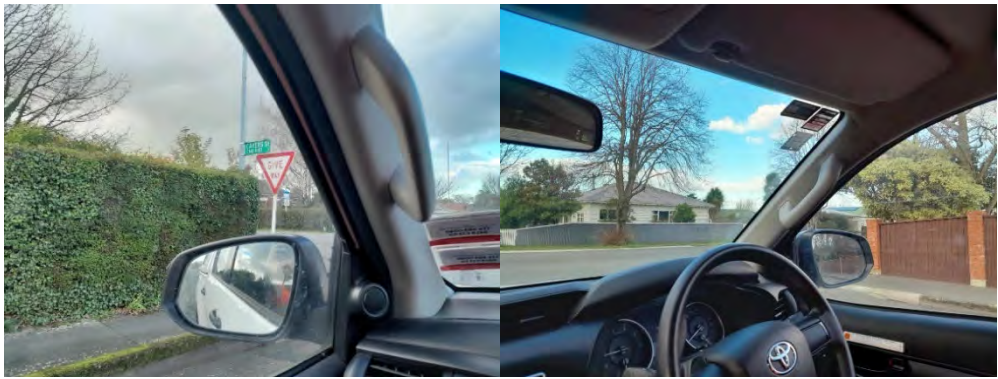
Figure 6. Visual of sight distance available at the Seddon Street/Ayers Street intersection on the western approach.
