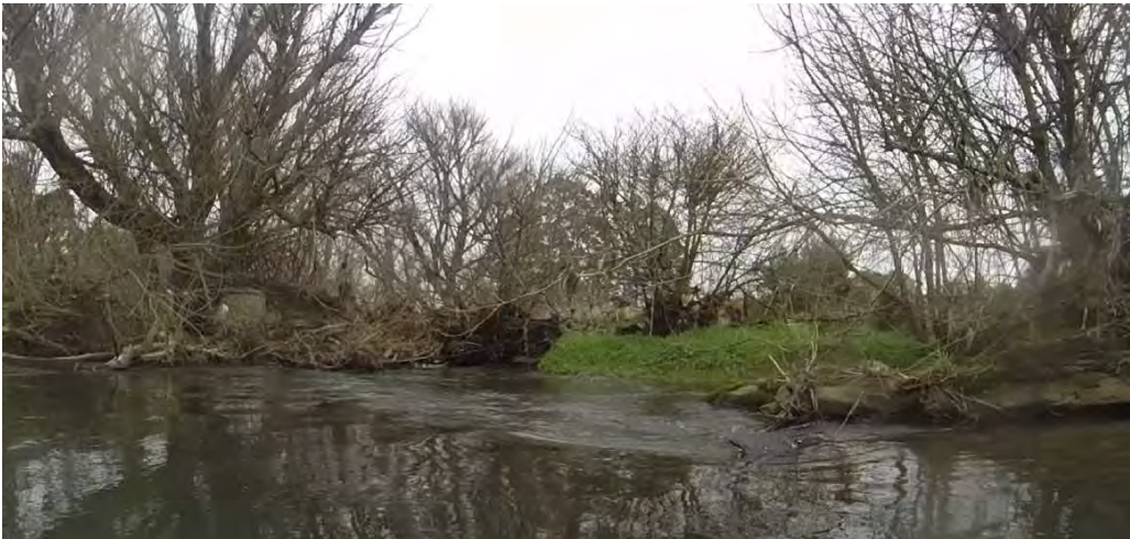
Figure 4 - Fallen tree debris observed on maintenance inspection.
