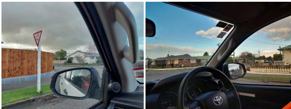
Figure 12. Visual of sight distance available at the Seddon Street/Ashgrove Street intersection on the western approach.
