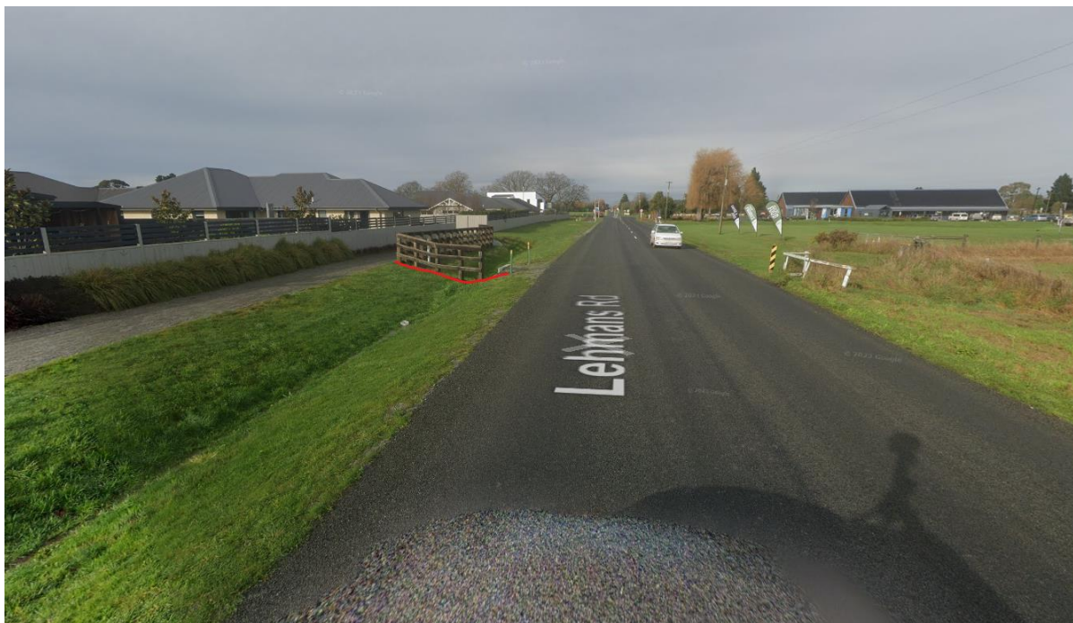
Figure 8 Current Lehmans Road swale drain (adjacent to Westpark)
