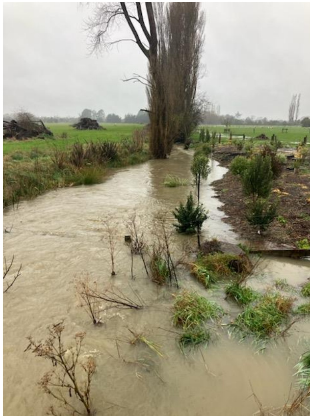
Photo 6 – Unmaintained channel that was cleared 29/7/24
