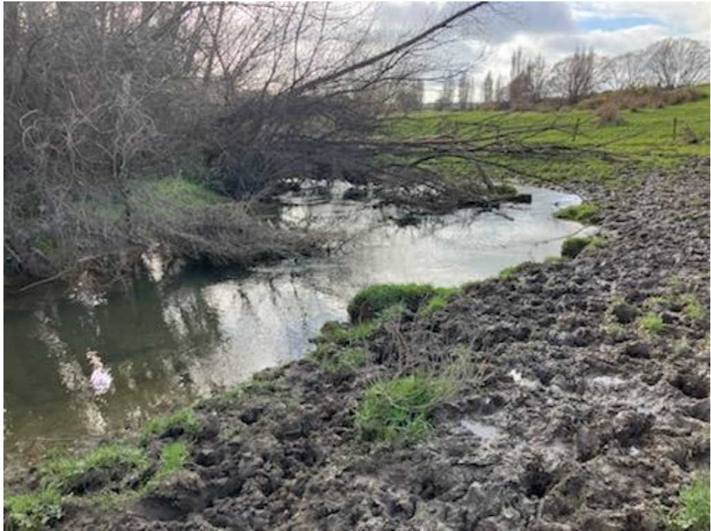
Photo 5 – Unmaintained drainage channels
