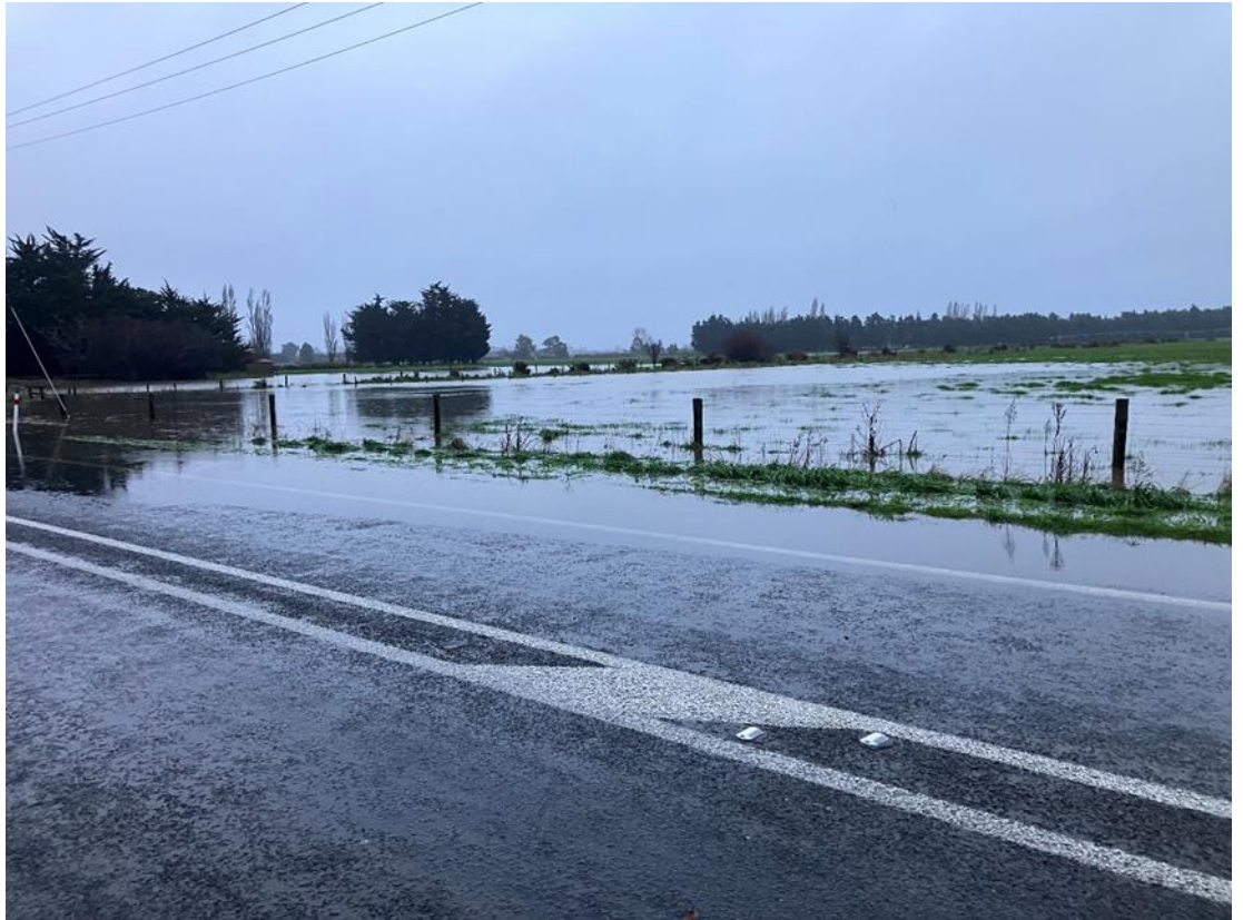
Photo 3 – Flooding in the proposed Eastern SMA area of the Site due to backwater from the culverts
