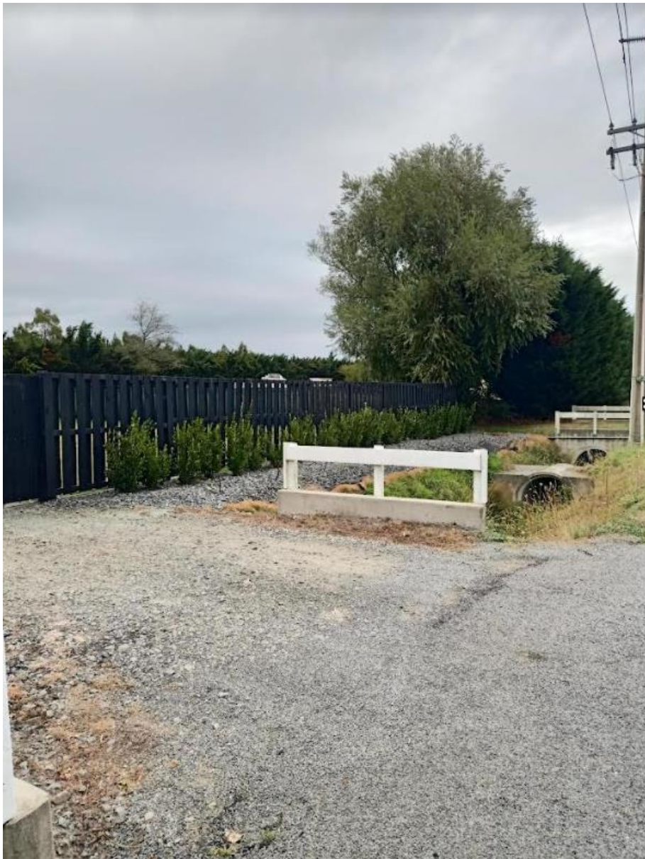
Figure 2: Existing vehicle crossing
