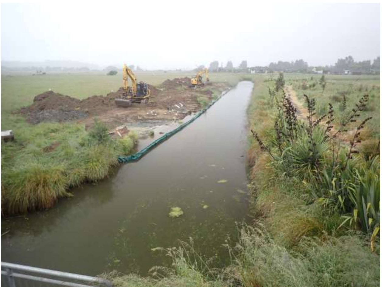
Figure 1: Rebatting earthworks on the True Right of the Taranaki Stream at the floodgate, for improved īnanga spawning habitat.
