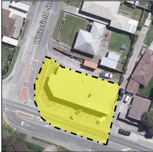
Ohoka Road Shops, Kaiapoi
