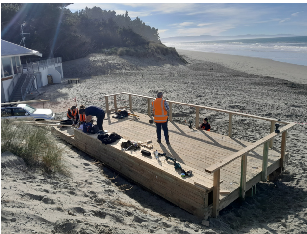
Progress on Waikuku Beach accessible platform
