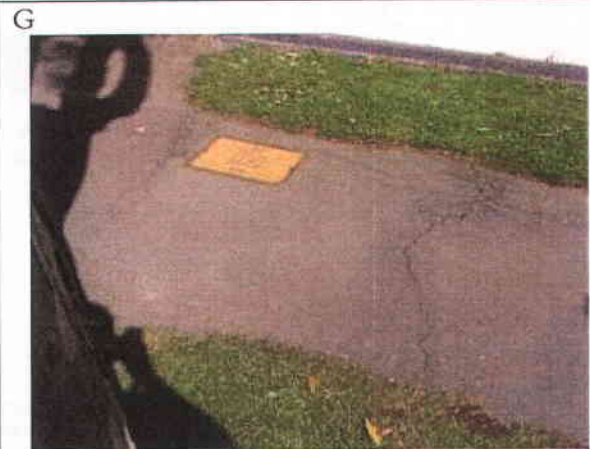
Frames F and G above show trees #19 and 22 respectively and illustrate two types of damage present in Queen Street. #19 has a series of cracks and raised Tarmac close to the tree; these were most likely caused by large lateral roots. Tree #22 shows cracks which are much smaller. Both areas of damage seem to be associated with civil engineering disturbance to the path.
