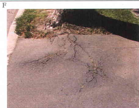
Frames F and G above show trees #19 and 22 respectively and illustrate two types of damage present in Queen Street. #19 has a series of cracks and raised Tarmac close to the tree; these were most likely caused by large lateral roots. Tree #22 shows cracks which are much smaller. Both areas of damage seem to be associated with civil engineering disturbance to the path.
