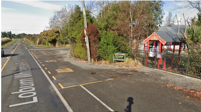
Figure 1. Existing bus stop
