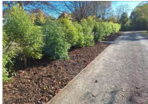
Completed Wilson Drive Stormwater Upgrade
