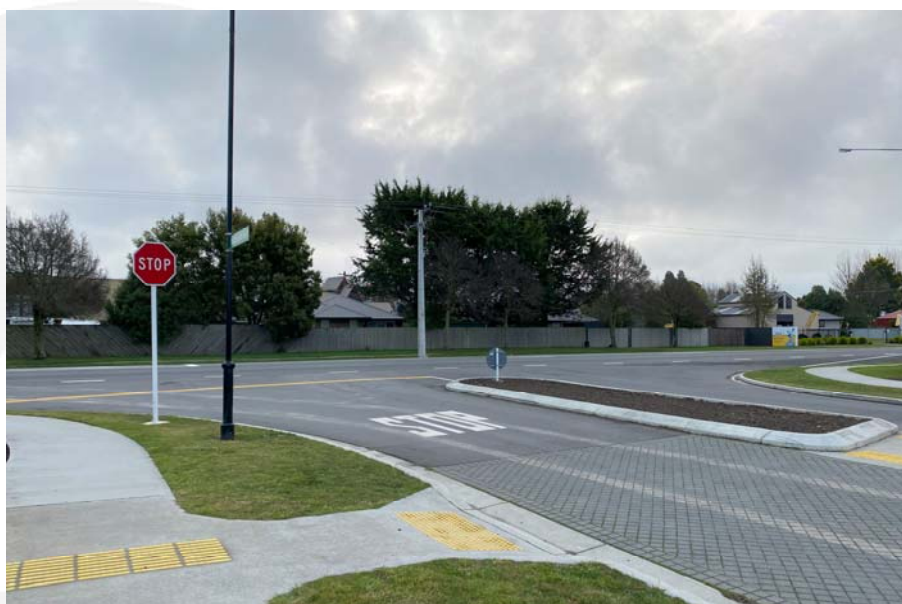
Photograph 8: Main North Road / McQuillan Avenue Intersection Looking Northwest
