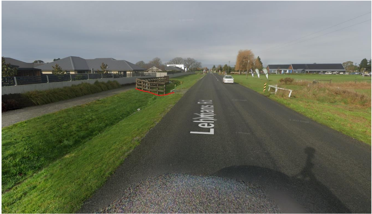
Figure 12 Current Lehmans Road swale drain (adjacent to Westpark)
