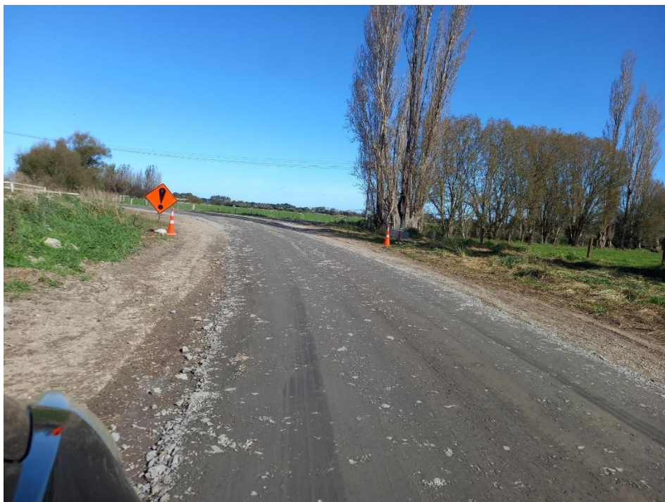
Figure 7: A trial argillite roading section on Waikoruru Road, in the approach to the bridge over the Cam River. Note the argillite has created a hardened surface that prevents erosion of the material and dust into the waterway.
