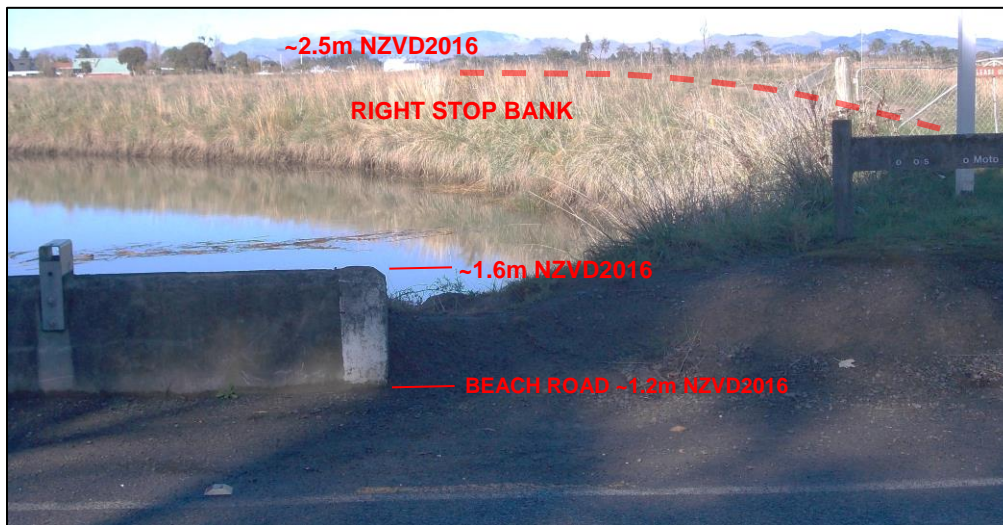
Figure 21: Beach Road bridge crossing on Kairaki Creek, looking downstream (10 May 2019)
