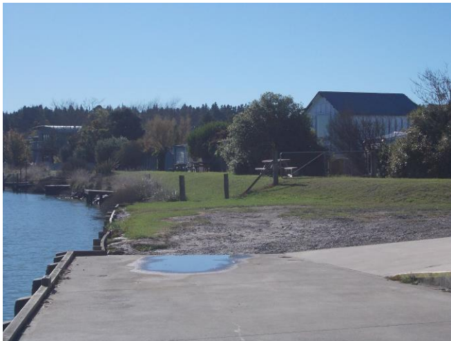
Figure 2: Kairaki Creek, left bank at Sailing Club
