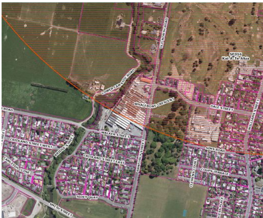
Figure 1: Silent file area 'Te Kai a te Atua' (red circle) upstream of the Cam River flood gate structure.
