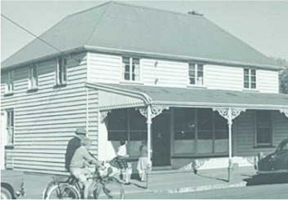
Building before ground floor modification and installation of shutters. www.
