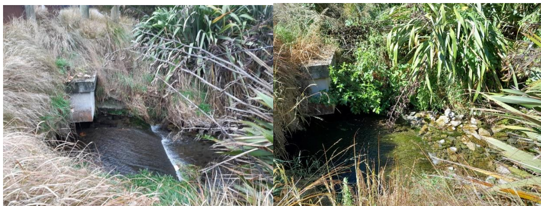
Figure 2: The likely fish passage barrier on a North Brook tributary – Corner of Cotter Lane and Northbrook Road before (left) and after (right) works were carried out
