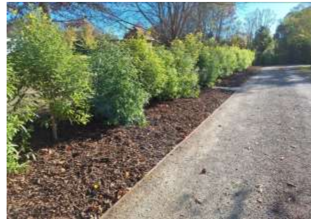
Completed Wilson Drive Stormwater Upgrade
