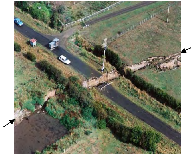
a) Edgecumbe Fault – The 1987 Edgecumbe earthquake resulted in about 7 km of surface rupture along the Edgecumbe fault, and up to about 2 m of vertical displacement of the ground surface at the fault (Beanland et al 1989). Arrows mark the location of surface fault rupture.
