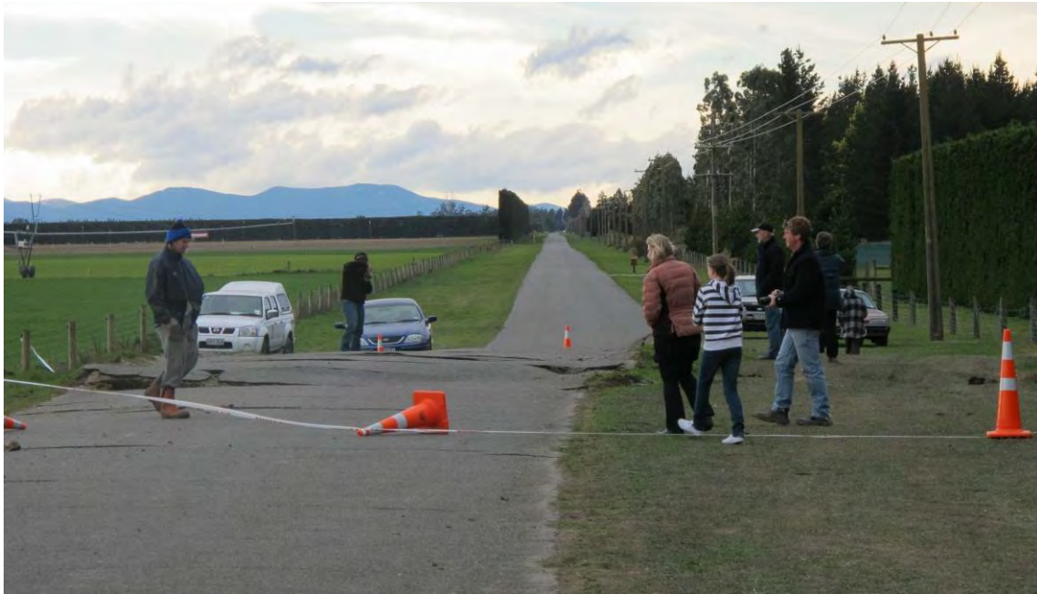
Figure 1.2 Surface fault rupture on the Greendale Fault at Highfield Road in Selwyn District (see Figure 1.1 for location) during the 4 September, 2010, Darfield (Canterbury) Earthquake. Before the earthquake, the road was straight and the ground was flat. At this location, surface fault rupture formed a ~40 m wide zone of fractures and broad folds in the ground resulting from mostly sideways ('strike-slip') ground shift of ~4.5 m. In addition, the south side (near the camera) was bulged up by about 1 m. Photo: D.J.A. Barrell, 5 September 2010.
