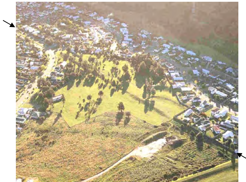
a) Wellington Fault at Totara Park.
