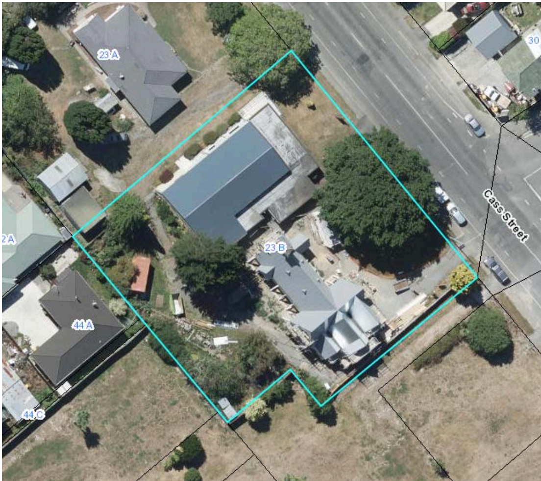
Extent of setting, St Bartholomew's Anglican Church, 23B Cass Street, Kaiapoi.
