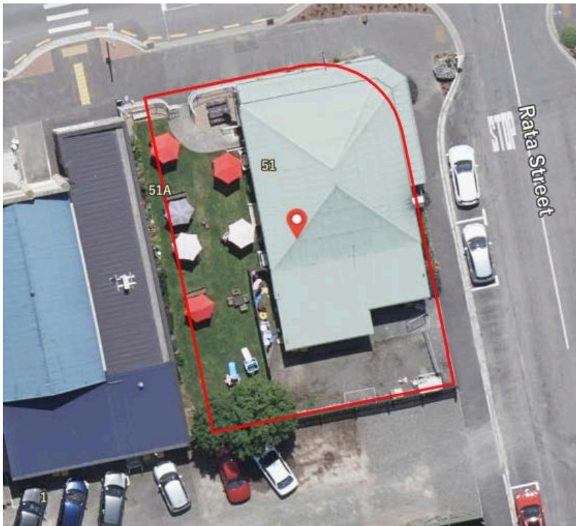
Extent of setting, including the road reserve over which the veranda projects, 51 Main Street, Oxford.
