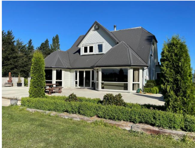
Dwelling 2 – relocated to site post-earthquakes
